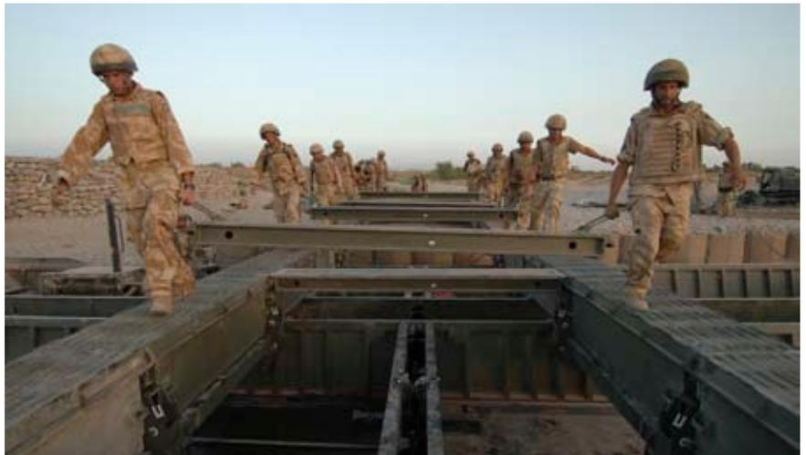
*In an operational engineering first, engineers lay an air portable ferry bridge across the River Helmand in just seven hours*
